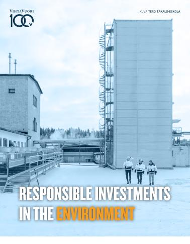
Several environmental investments have been made in Vihtavuori over the years, such as improving waste heat recovery and energy efficiency and reducing water use. Two of the factory's cooling water circuits were turned into closed circuits in 2016–2019. Waste heat is recovered from these cooling circuits with heat pumps, and this energy covers 20–30% of the energy needs of the entire factory. Thanks to the change, the plant now uses 50% less water than before.
